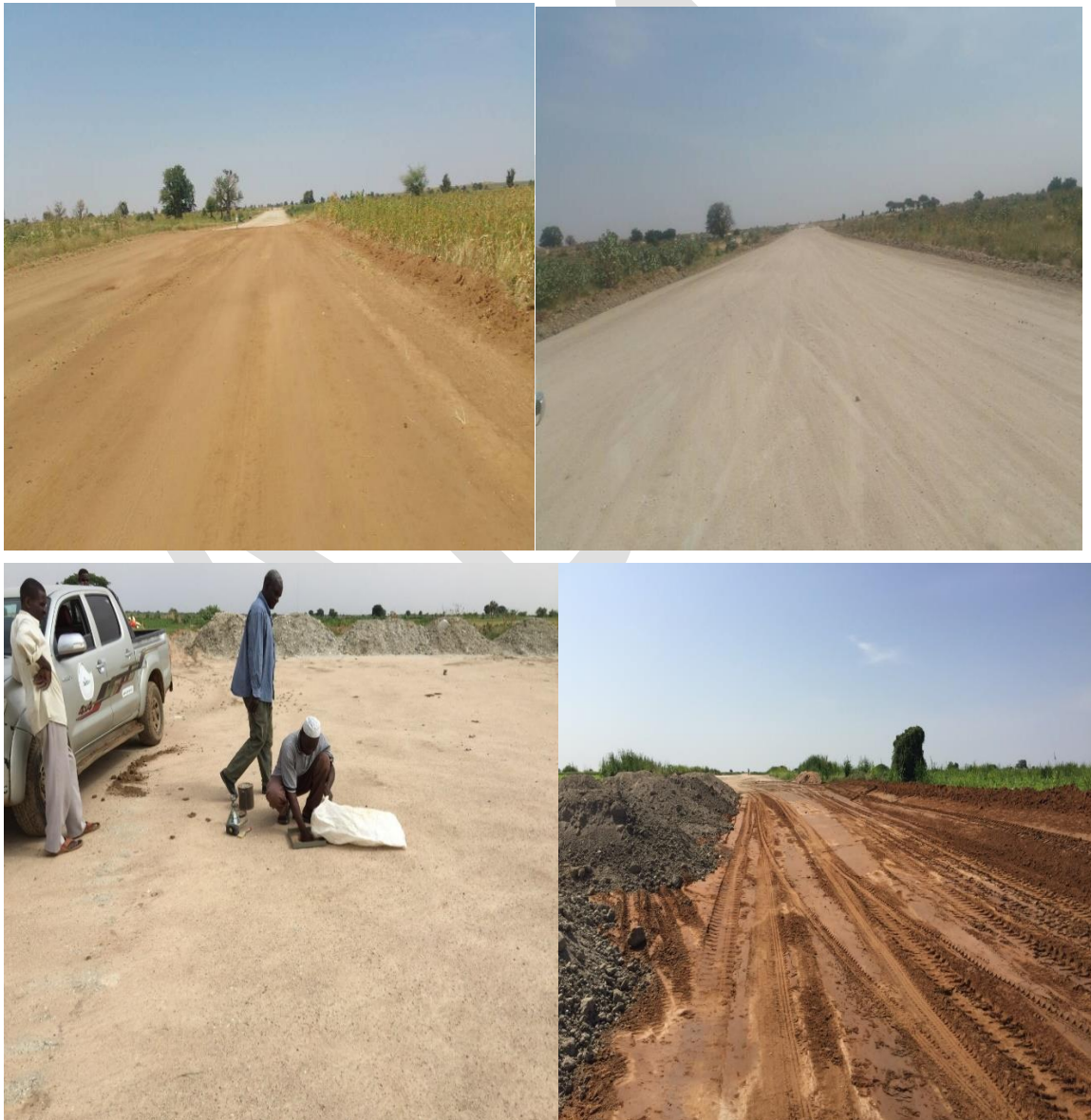
Figure6: Images from Nyala – Geraida – Buram Road (Phase one 42 km) Project – Embankment Work (First Layer)
